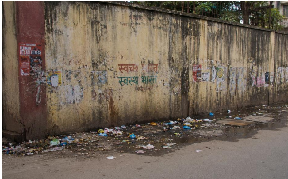
Figure 2: Visual evidence of public defacement and spitting on city walls.
